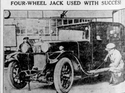
The four-wheel jack is now being used in England with much and much blessing from motorists. The four jacks are placed under axles next to all four wheels, and by means of a pumping handle on running board of the car, the entire machine is lifted from the ground. jack handle is easier to use than a bicycle pump.
