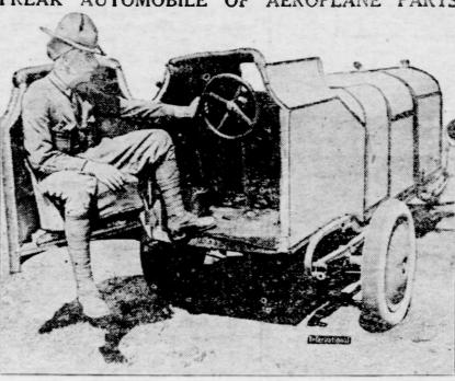
This freak automobile is designed and owned by a United States army man stationed at Mitchel field, Long island. It is built entirely of airplane parts and all driving and manipulation of gears is done from the stearing
