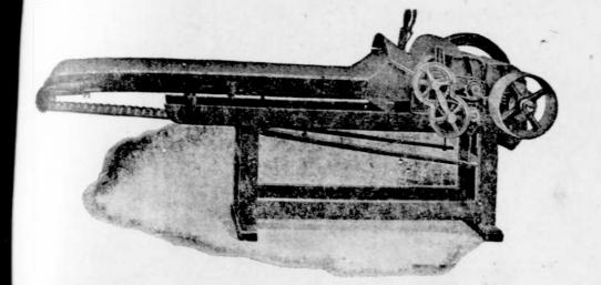
Self-Feed-This feature consists of a traveling feed chain, made of heavy iron slats ited to a chain which passes over the lower feed roller. Throw the fodder into the the "Plymouth" does the rest.
