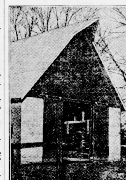
A Permanent Concrete Crib.
