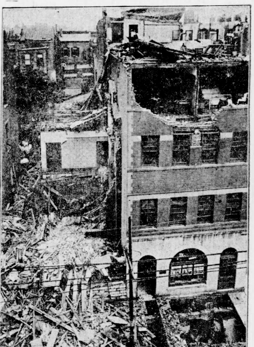
One of the many buildings wrecked by the furious wind and rain storm that did more than a million dollars' damage and killed about thirty persons in Cincinnati.
